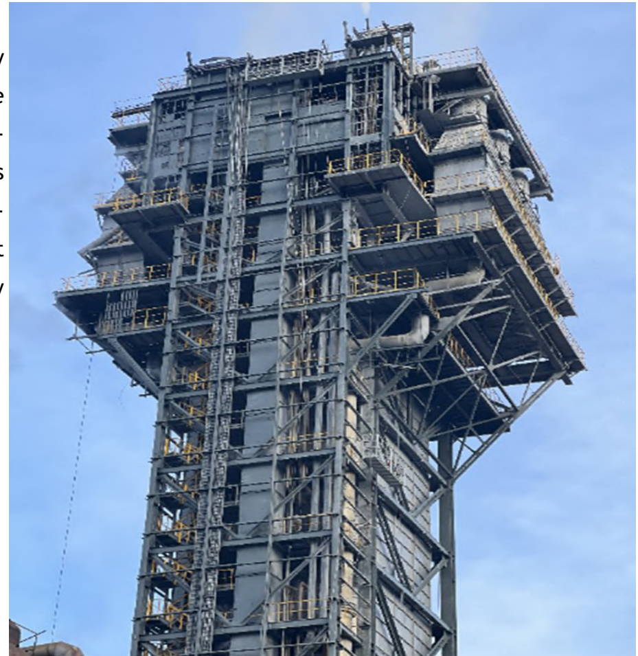
JSC Rustavi Azot Ammonium Nitrate Prilling Tower
